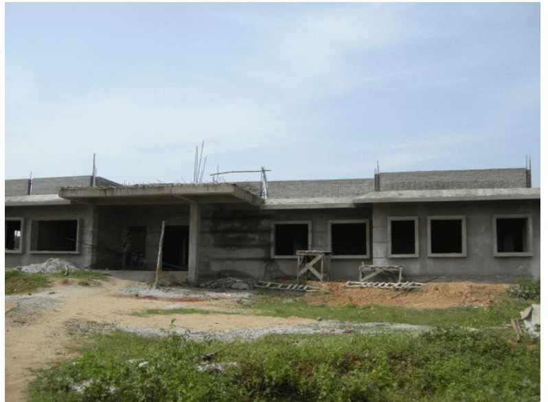
Chaminade Health Center
